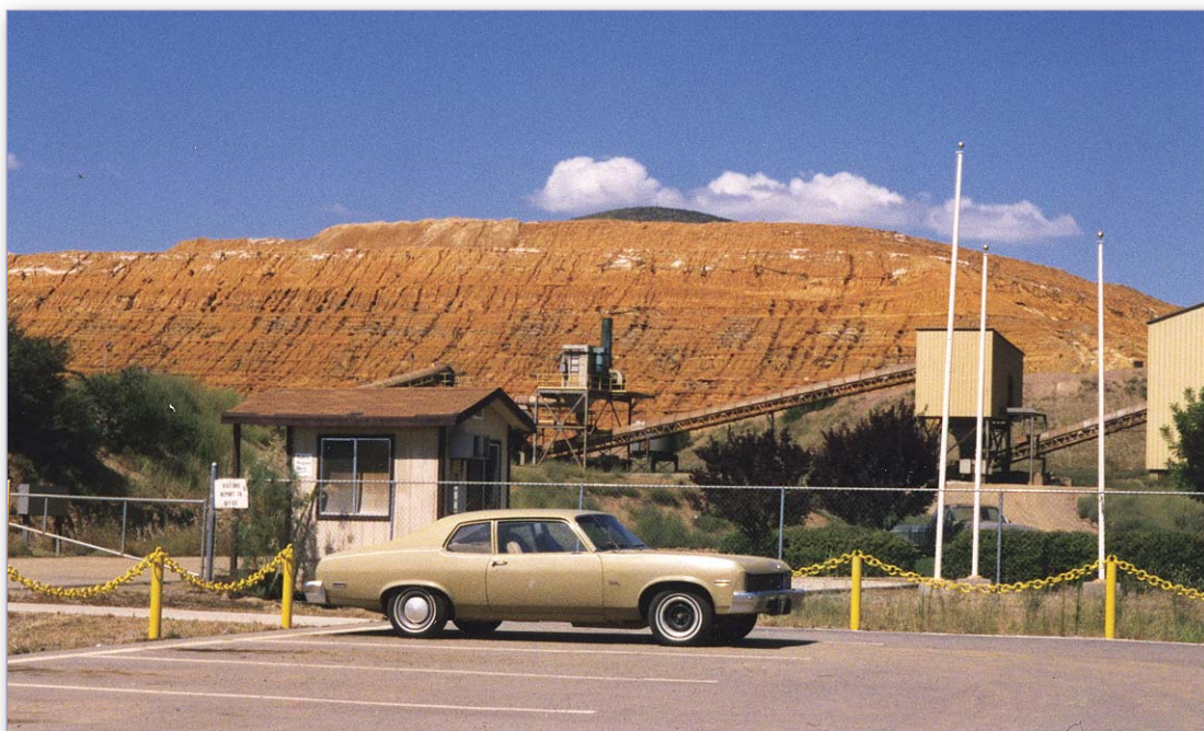
The Ironite facility at Humboldt, AZ. The orange mountain in the background is the pile of mine waste from which Ironite is derived.
